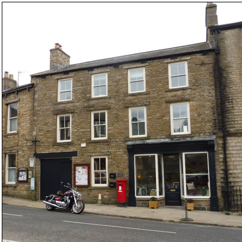
Askrigg Foundation where three affordable dwellings were recently completed by converting the upper floors and an outbuilding
